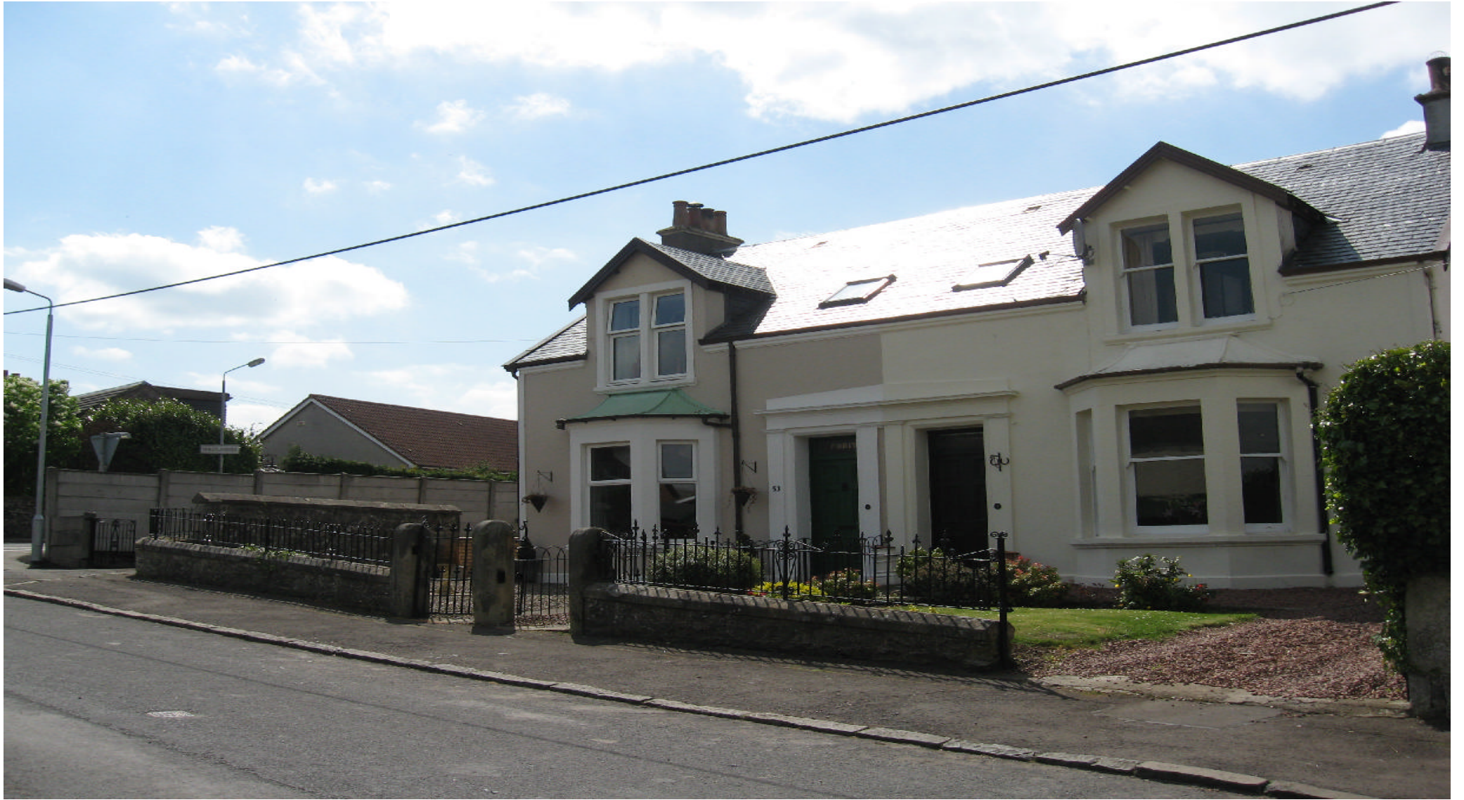
(Photo A) Front Elevation of host dwellinghouses
