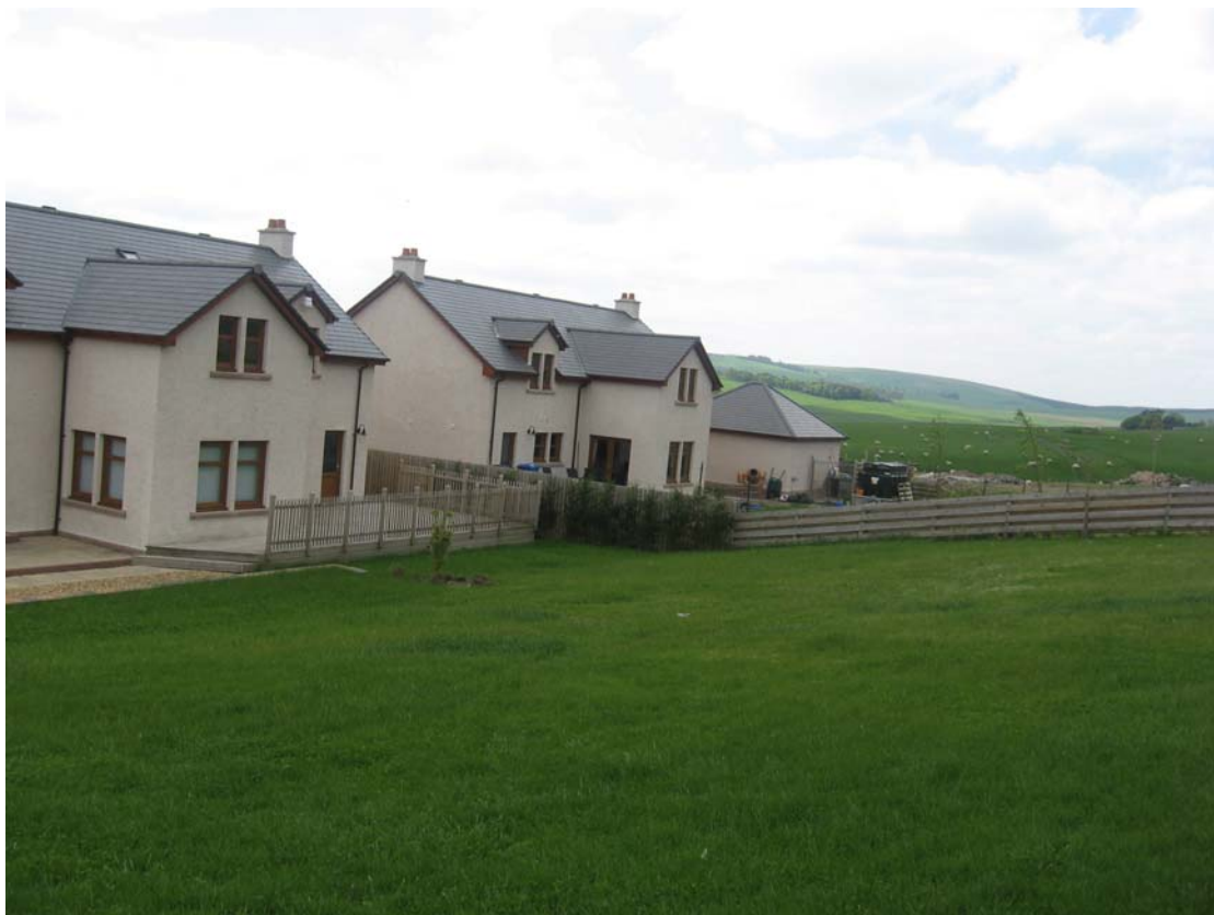
Photo 10 Timber fencing between numbers 1 and 2 West Millrigg.
