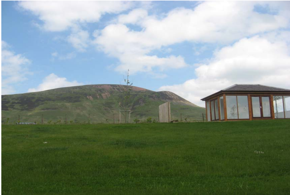
Photo 7 Glazed garden building and 1.8 metre screen fence.
