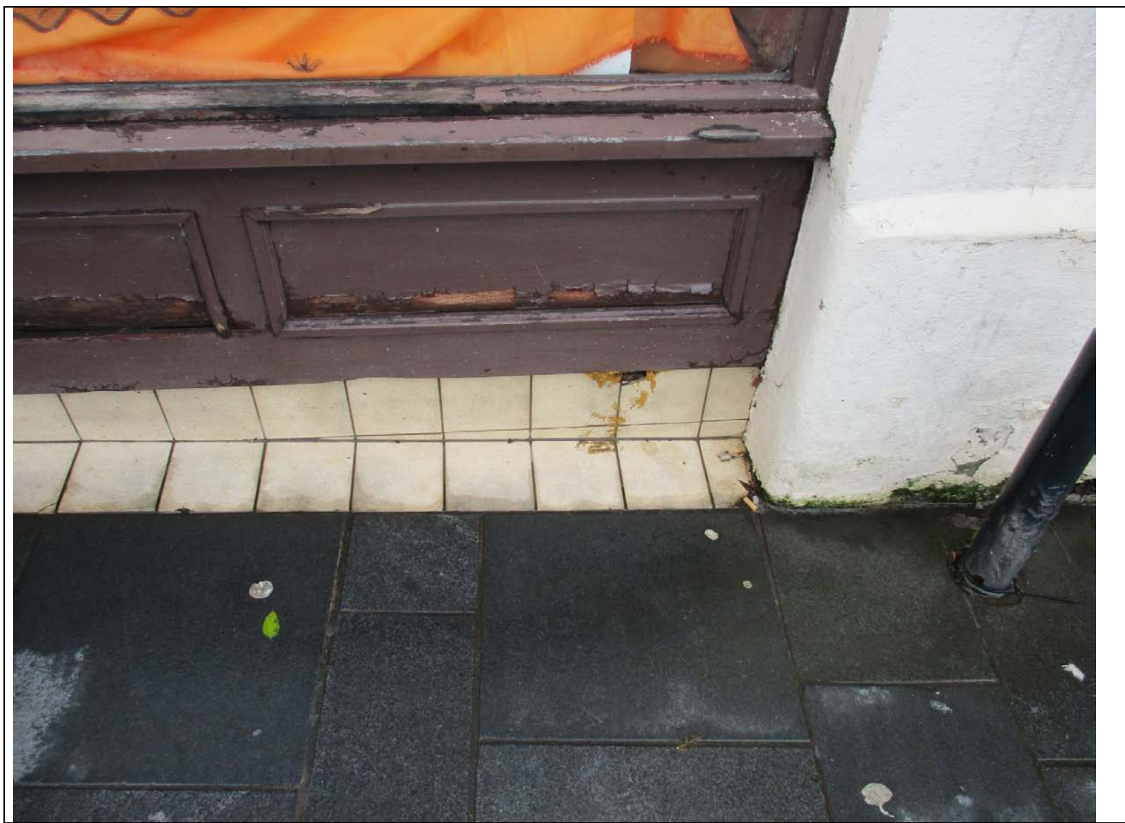
Photo 8 - Timber paneled stallriser ( taken 12/10/2017)
