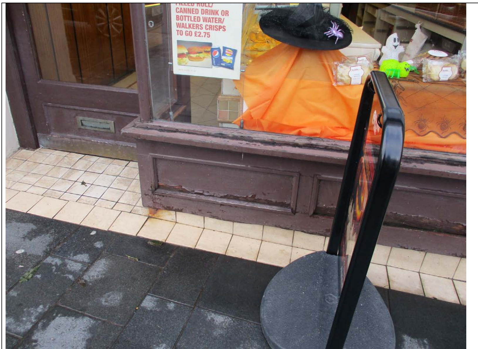
Photo 7 - Timber paneled stallriser ( taken 12/10/2017)
