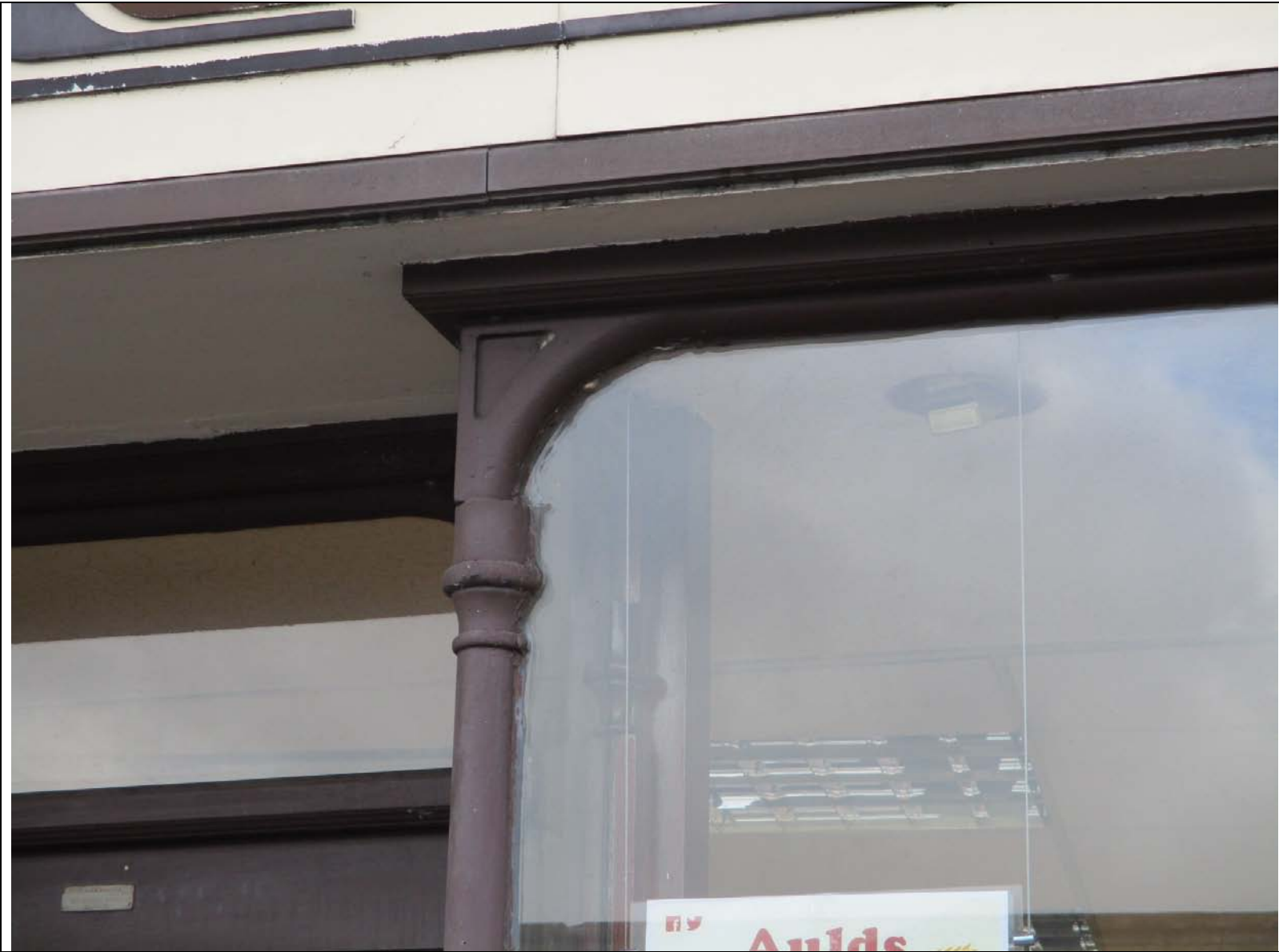
Photo 4 – Curved window detail ( taken 12/10/2017)
