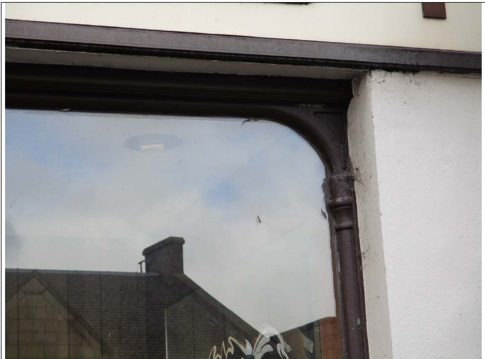
Photo 5 – Curved window detail ( taken 12/10/2017)
