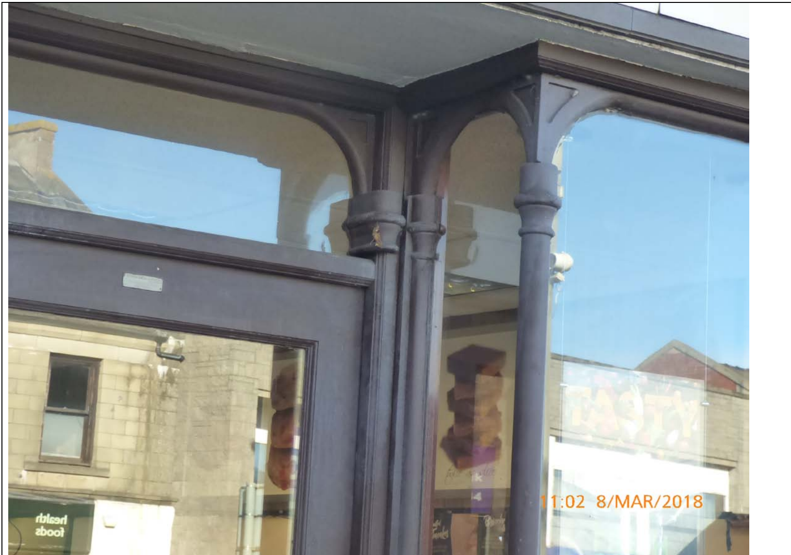
Photo 3 - Curved fanlight and window details with turned wood detailing.( taken 8/03/2018)
