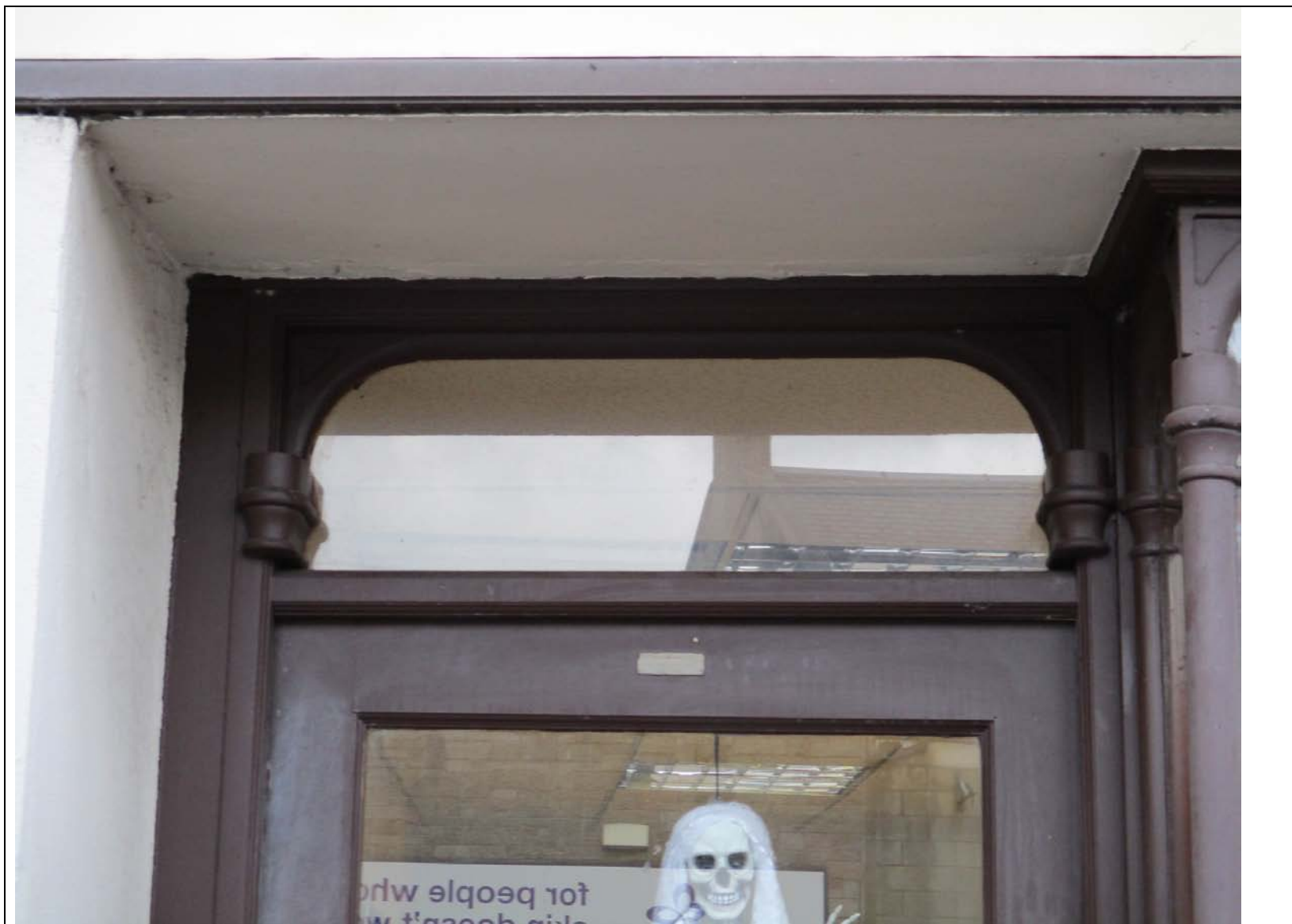
Photo 2 – Curved fanlight above door( taken 12/10/2017)
