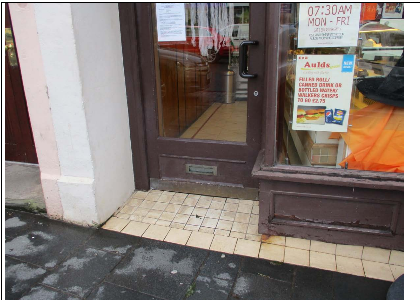
Photo 6 - Tiled entranceway, timber door with kickboard and timber paneled stallriser ( taken 12/10/2017)
