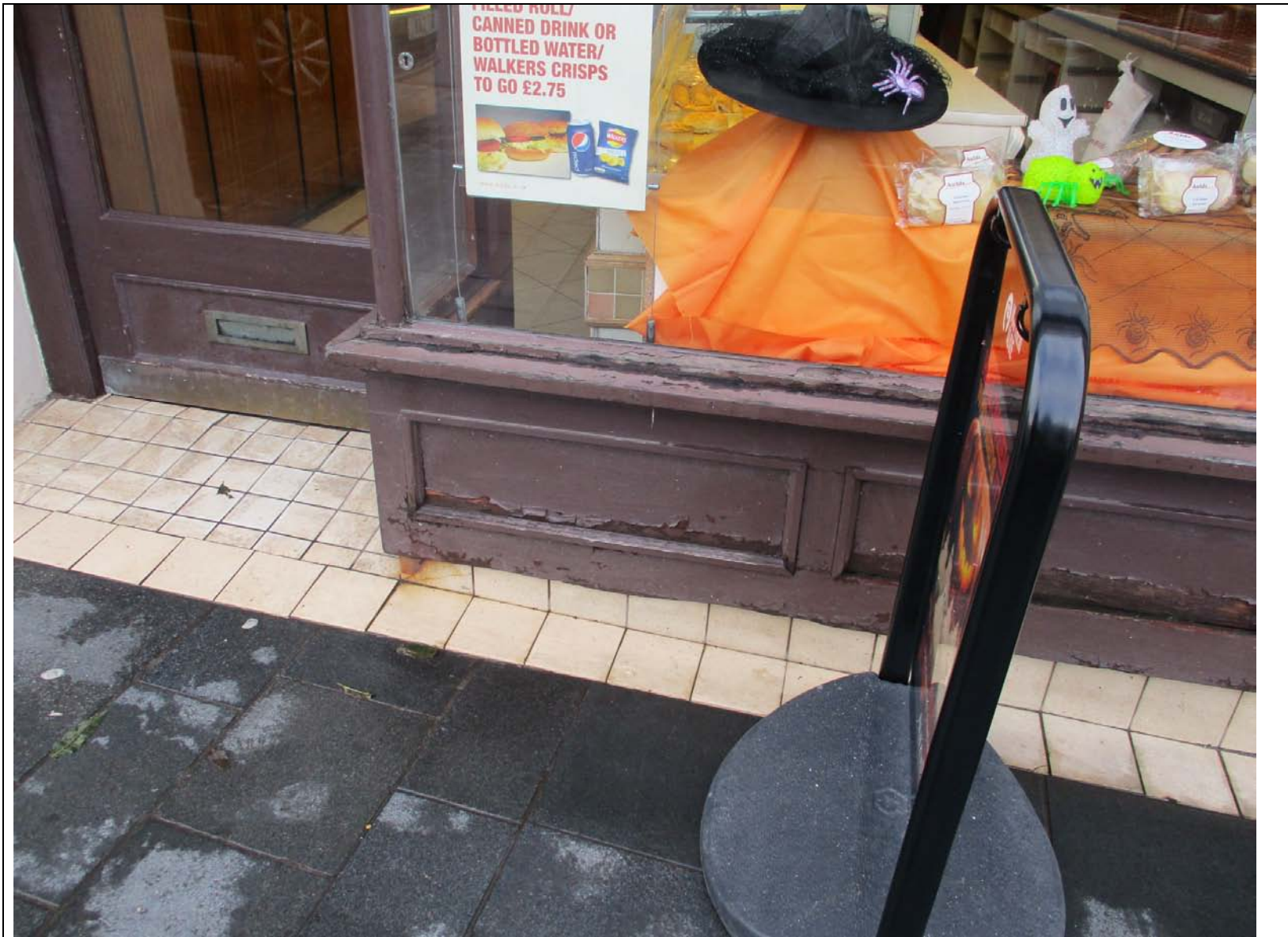
Photo 7 - Timber paneled stallriser ( taken 12/10/2017)
