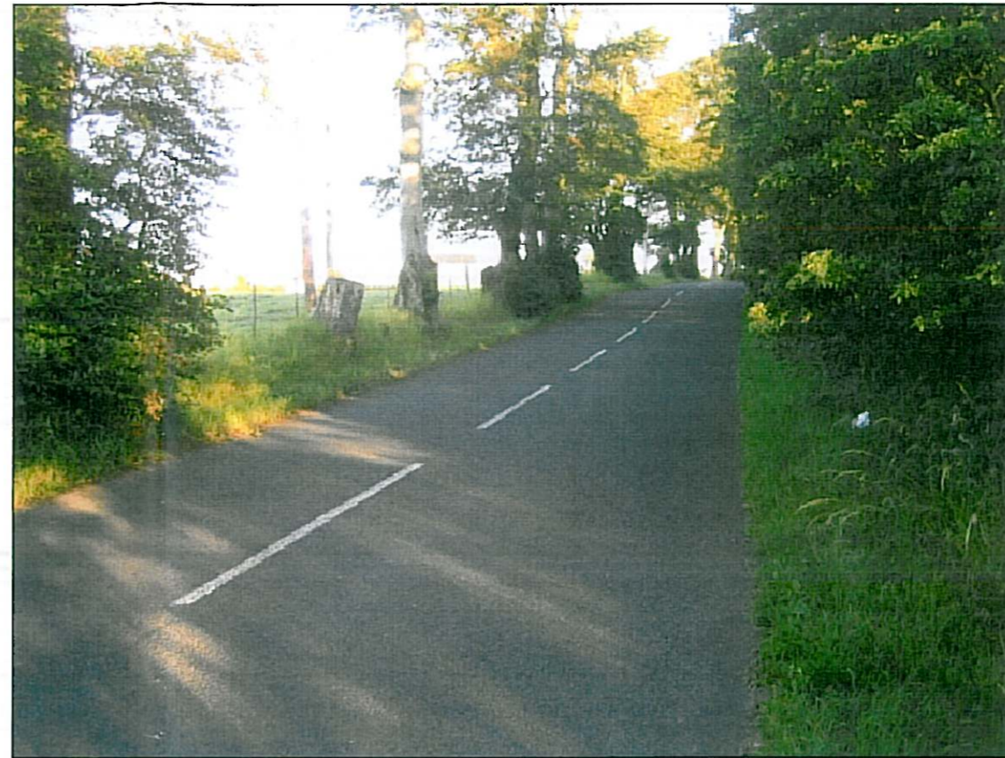
PICTURE 2 — LOOKING WEST FROM THE EXISTING SITE ENTRANCE
