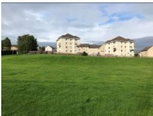
Local Authority Blocks on Fleming Way
