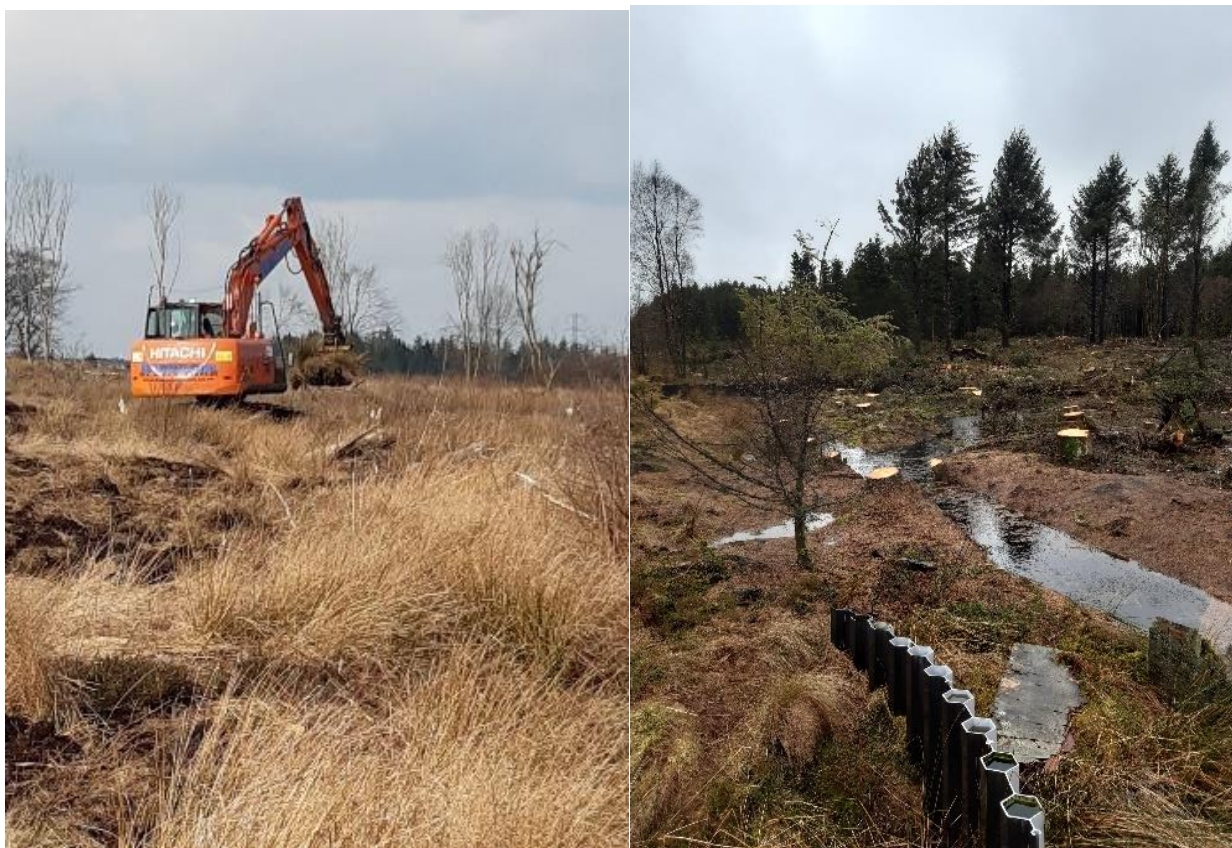
Photo 10: Contractor installing peat dams at Langlands Moss LNR.
